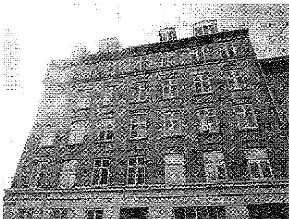
Overfacade mod gade
