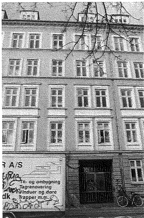
Facade mod gaden
